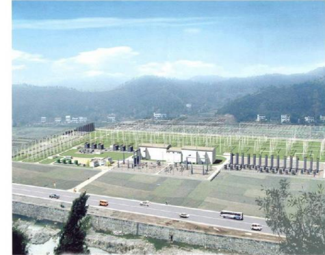
HVDC Converter Station 1000 - 12000 MW, Classic
